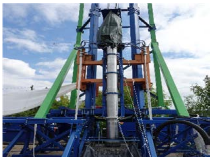
Figure 1: Mounted drill hammer with pipes for drilling fluid
